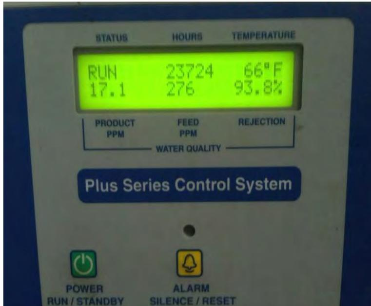
93.8% rejection which is close to the rejection percentage when the membrane is new
