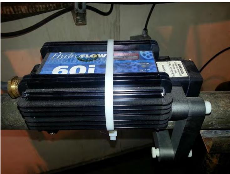
HydroFLOW 60i placed on water line feeding the RO system
