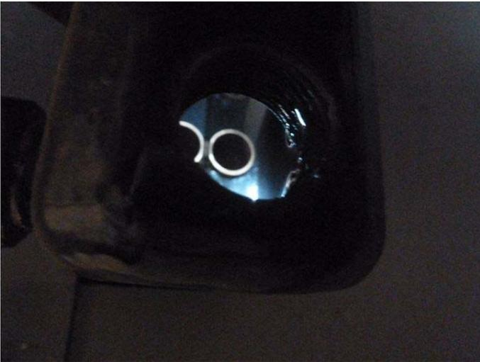
Heat exchanger tub viewed through inspection port. Absolutely NO SCALING was observed
