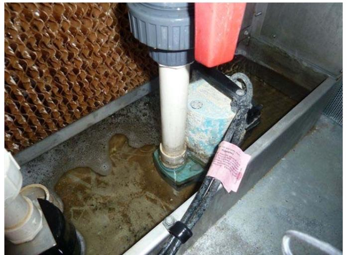
Pump and evaporative pad. Scale on the pump is from the previous season. Observe ALL SCALE below the water line is gone. Also observe pad is clear of scale build-up.
